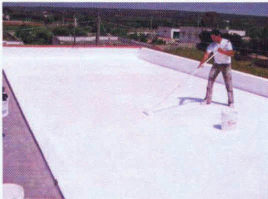
White paint on a flat roof
