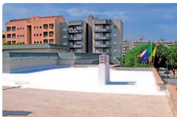
Figure 14. View of the roof with a partial application of the cool roof paint
